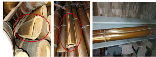
Fig. 9. Collapses occurred in the middle of the bamboo poles.
