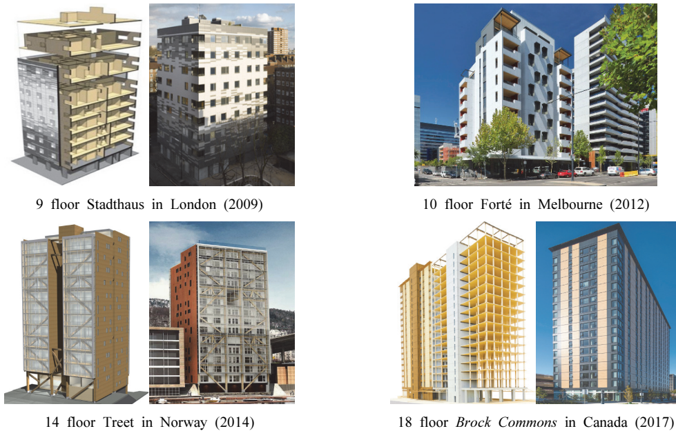
Fig. 2. CLT buildings (Xiong et al. , 2016; Li et al. , 2019; Malo et al. , 2016; Fast et al. , 2016).
