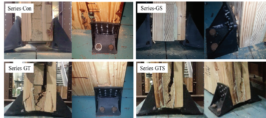
Fig. 5. Failure modes of the uplifted CLT connections under monotonic loading.
