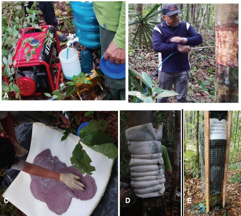
Fig. 2. Treatment of standing tree using a combination of injection (above) and bandage-wrapping methods (below); preservative injection is applied to the tree stem under pressure. A: preparation of preservative solution; B: injection of preservative solution into the living tree using a pump; C and D: preservative solution for bandage-wrapping mixed with CMC (carboxymethyl cellulose) is applied to the living tree; E: Experimental trees protected with wire.
